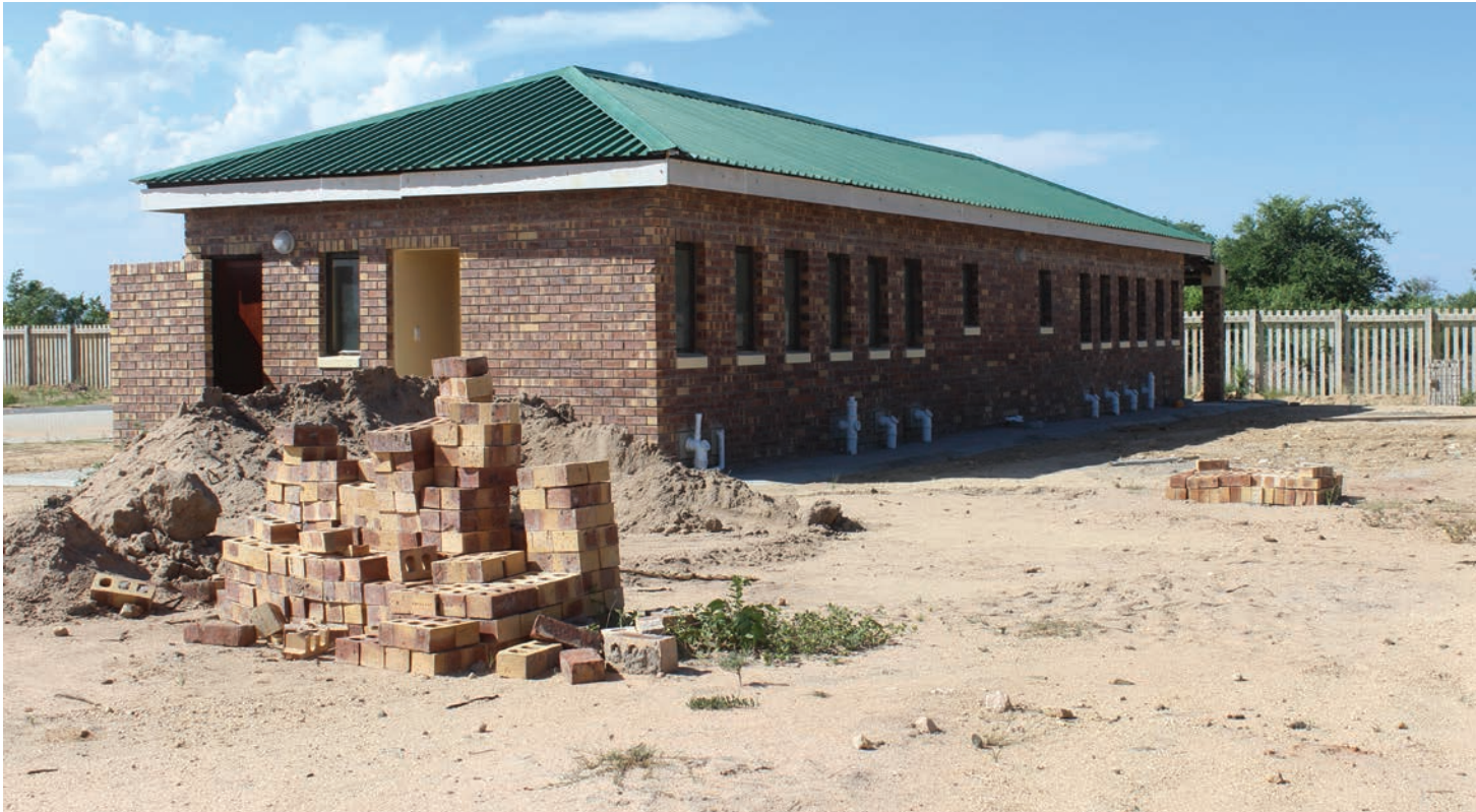
The Edinburgh landfill site – state-of-the-art ablution facilities under construction.
